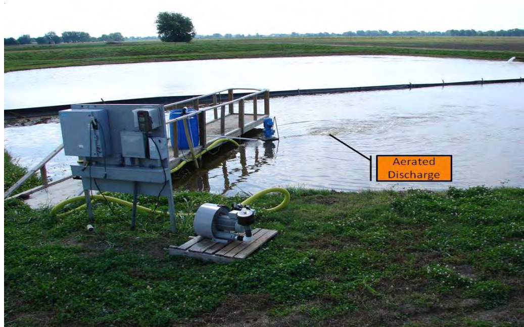
Figure 20. Prototype U-Tube with pond full. Discharge can be seen.
